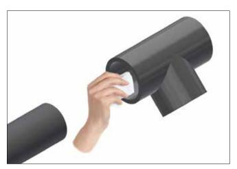
Pipes and fittings are cleaned with Griffon Cleaner. Apply detergent to a cloth. Clean and degrease surfaces. Remove any condensation and allow the surfaces to dry properly.
