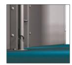
The gates are mounted on sloped hinges, so that they raise when opening. When closed the gates fit tightly to the floor and prevent manure in the aisle.
