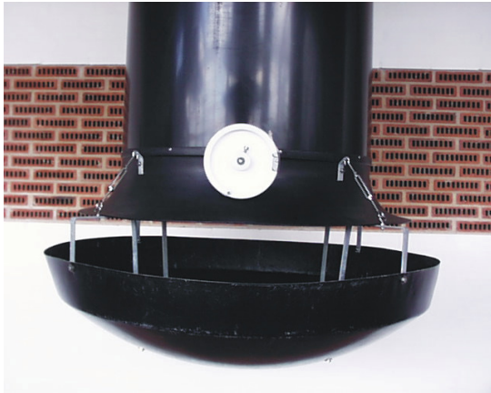
The light dimmer placed under the exhaust
